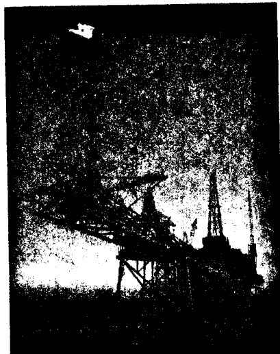
North Rankin A gas drilling platform, North West Shelf, 130km off Dampier, Western Australia
